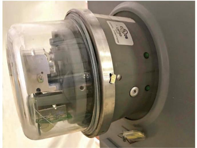
**New-Mac Electric has meter cans from two manufacturers currently installed. The Sycom meter can (above) is dark gray with green lights on the right side. The Tesco unit (at left and below) is light gray with red indicator lights. It is easier to check these lights after sunset. As seen below, in order to check these lights during the day, you may need to partially cover the lights with your hand into make sure the lights are lit.**
