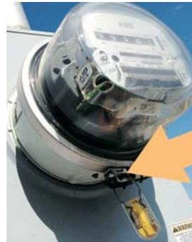
**The indicator lights need checked AFTER each storm has passed. These red lights will be lit if the device is still in working order.**
