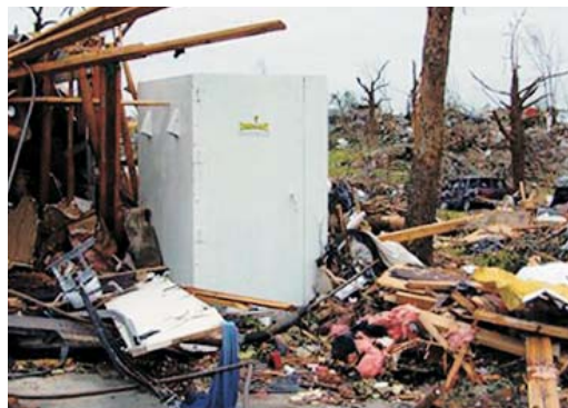
Another Twister Safe storm shelter that made it through the Joplin tornado
