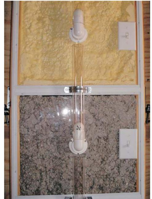
Among the energy-efficient applications New-Mac will have on display at the Newton and McDonald County Fairs are advanced framing methods (top left), a variety of types of insulation (above) and windows (bottom left).
